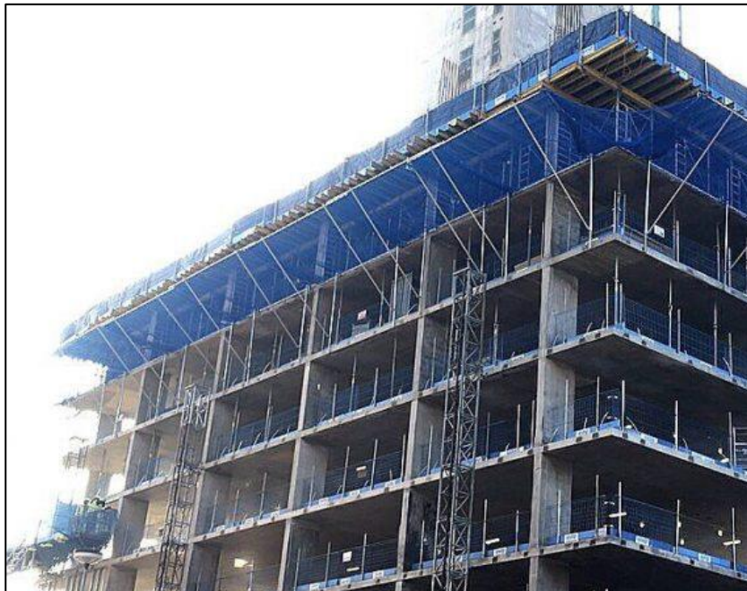
Figure 4-3: Example of Catch Platform
