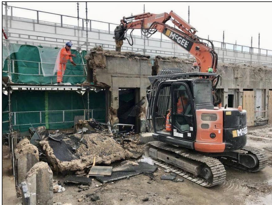
Figure 5-1: Top-Down Demolition Method – By Machine
