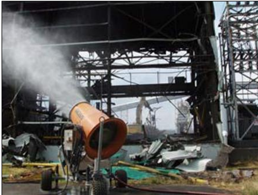
Figure 4-6: Example of Dust Control Using Water Mist System
