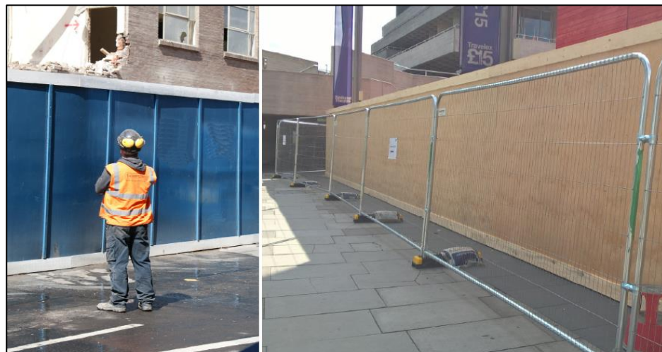
Figure 4-1: Typical Standard Hoarding Protection
