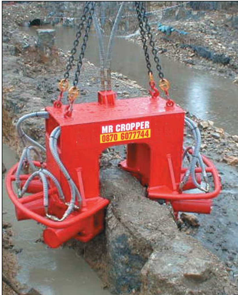
Figure 5-6: Pile Cutting/Demolition Method – By Hydraulic Crushing
