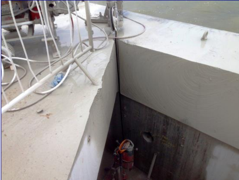
Figure 5-5: Wire Saw Cutting
