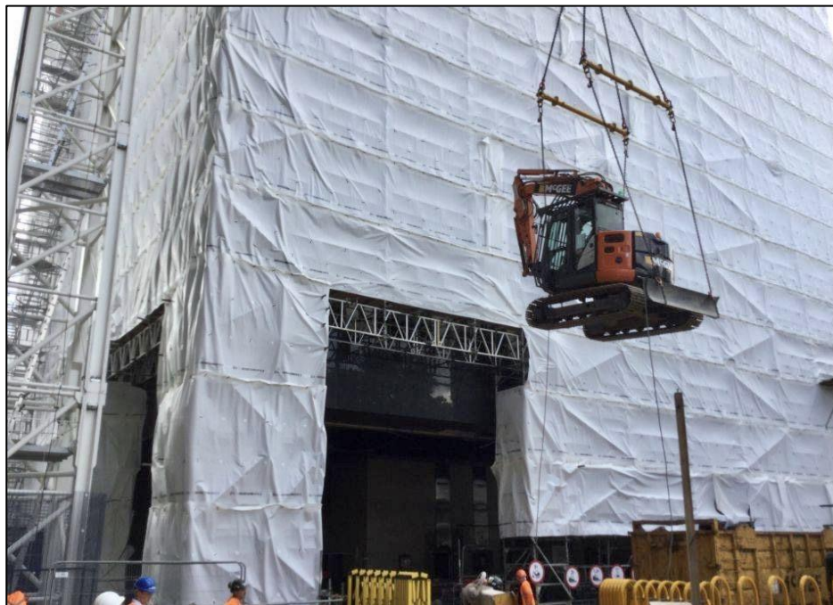
Figure 4-4: Example of Demolition Scaffolding and Screening
