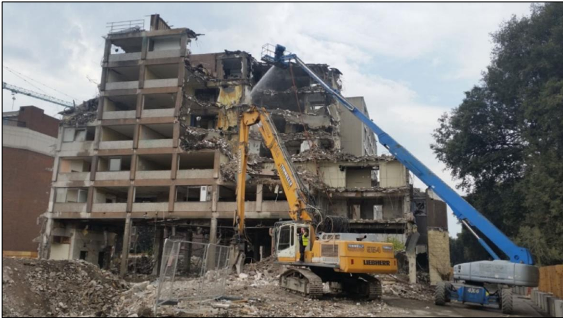
Figure 4-5: Example of Direct Dust Control by Damping Down
