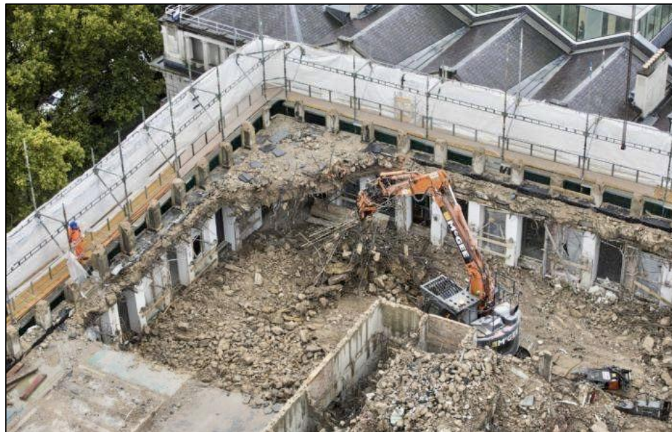
Figure 3-1: Typical Top-Down Demolition of Multi-Storey Building
