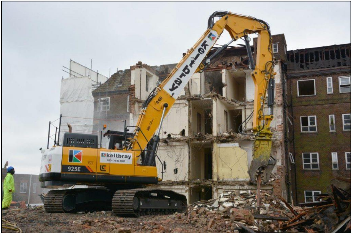
Figure 5-4: Top-Down Demolition Method – By Hydraulic Crushing Arm
